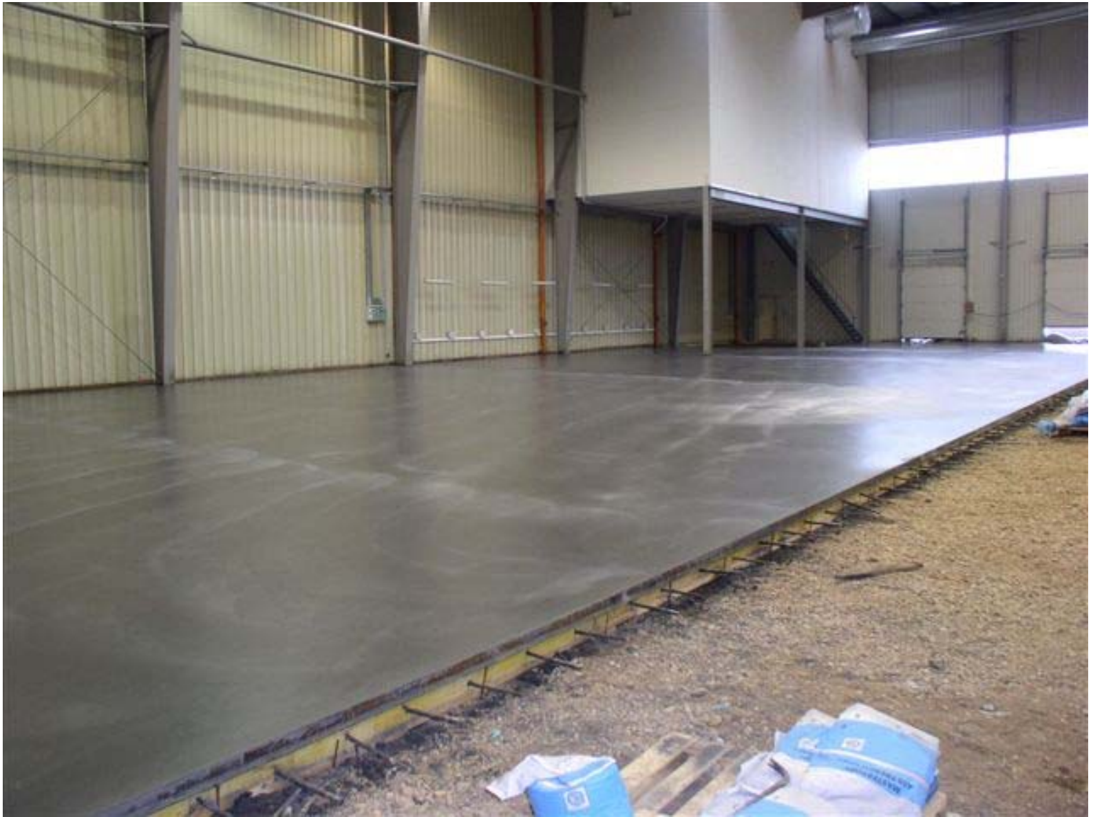
WAREHOUSE FLOOR reflects natural light after final polishing by regular discs.
